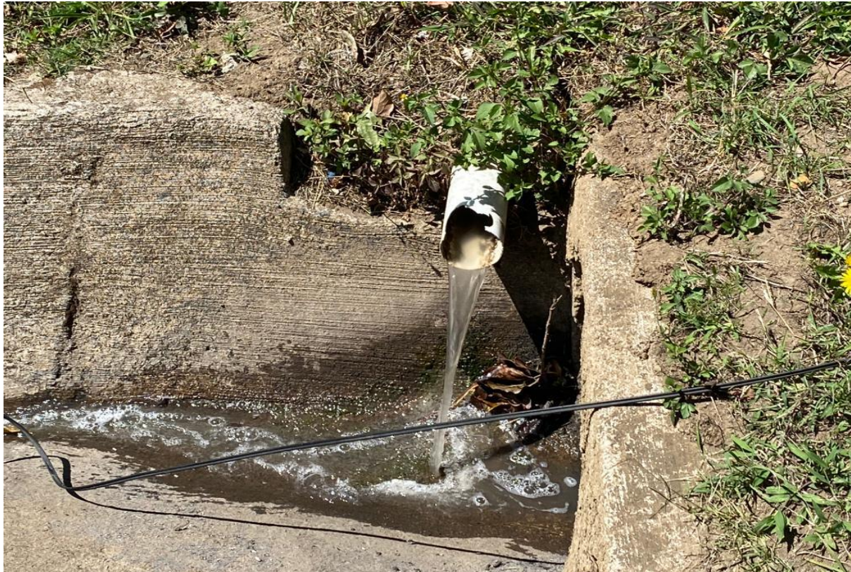
Greywater often goes untreated into the street
