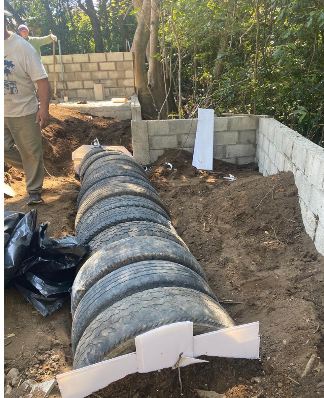
Modified septic tank using car tires
