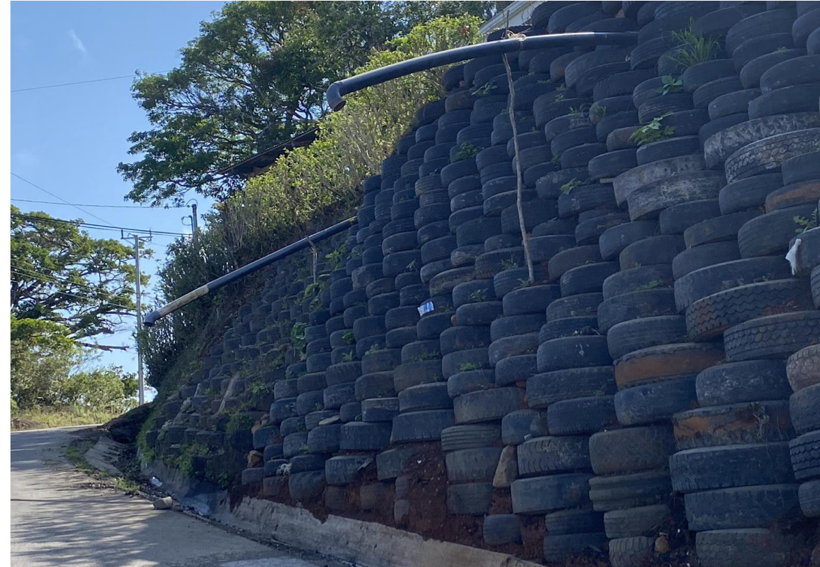
Greywater effluent discharging into the street
